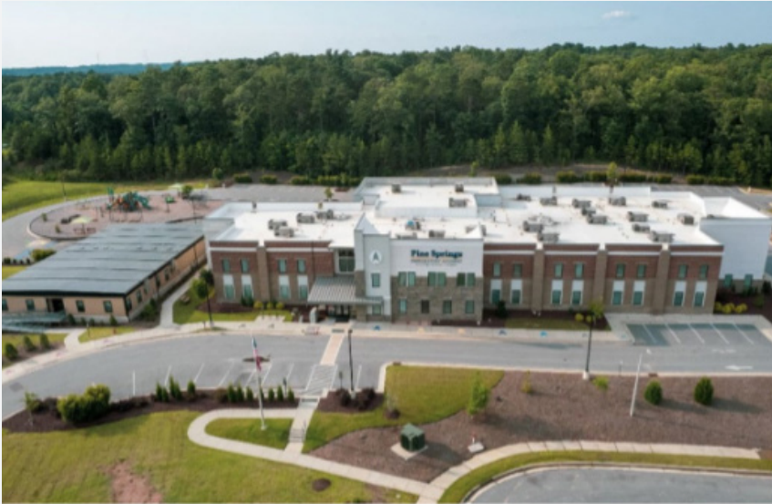
Pine Springs Preparatory Academy – Elementary School Campus
